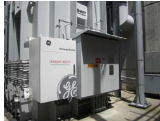
Cap Bank Impedance IED
