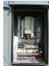
Cap Bank Impedance IED
