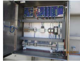
Cap Bank Impedance IED
