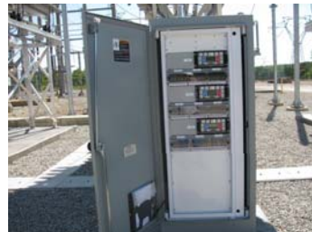
Cap Bank Impedance IED
