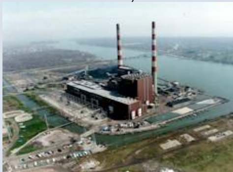
Trenton Channel - 730 mw
