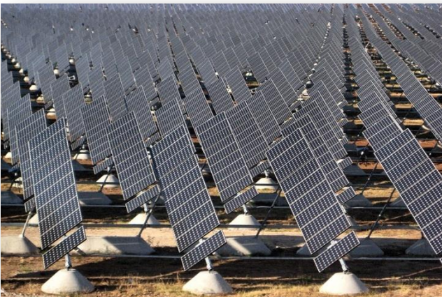
Olivenza, Spain 18 MW SunPower T0/T20 Tracker
