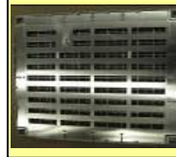
Perforated floor tiles with dampers
