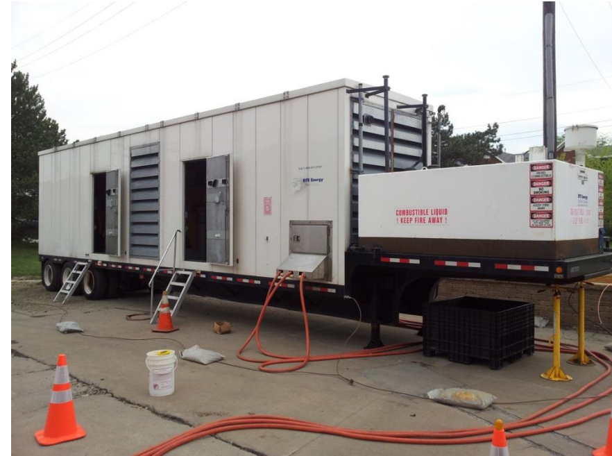
DTE 4.8 KV 1.5 MW portable generator
