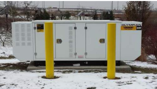
35 kW Natural Gas Generator
