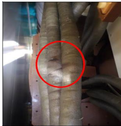
Photo 7 – Discolored Lead Paper Insulation
