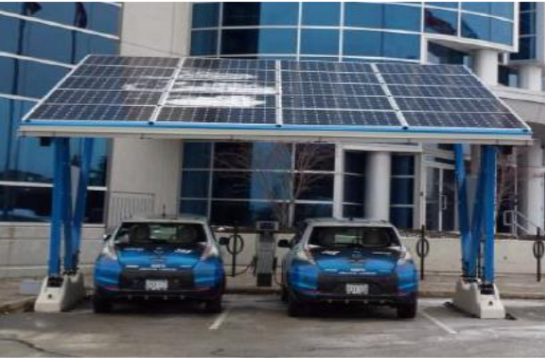
5 kW Solar Generator (EV Car Port)
