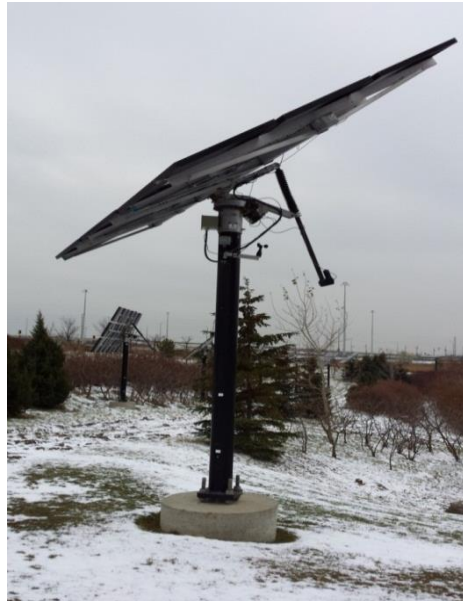
17 kW Tracking Solar Generator
