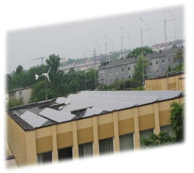
180 photovoltaic panels (250W) divided into three sections
