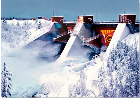
The Akkats hydro power plant (Lule river)
