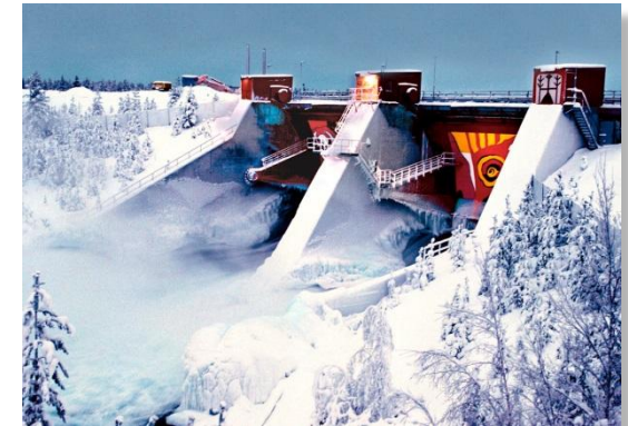
The Akkats hydro power plant (Lule river)
