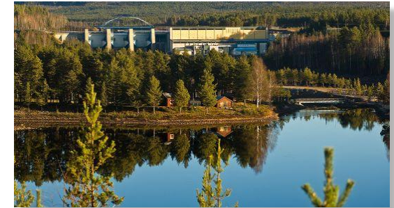
The Laxede hydro power plant (Lule river)
