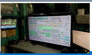
PI ProcessBook display on a 60in monitor to replace the magnetic board
