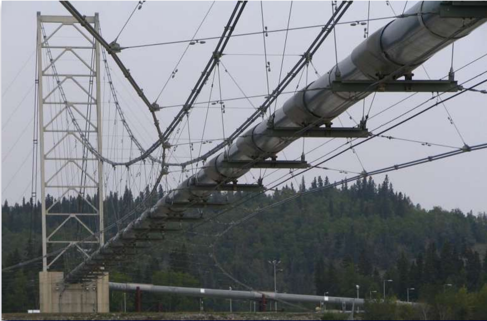
Tanana River Bridge Crossing
