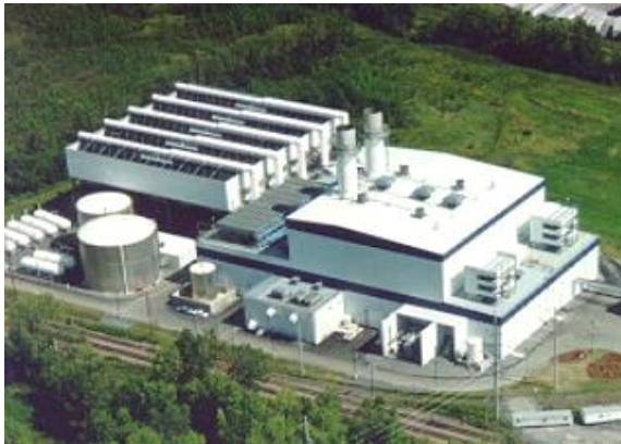
Air Cooled Condenser at remote Power Station
