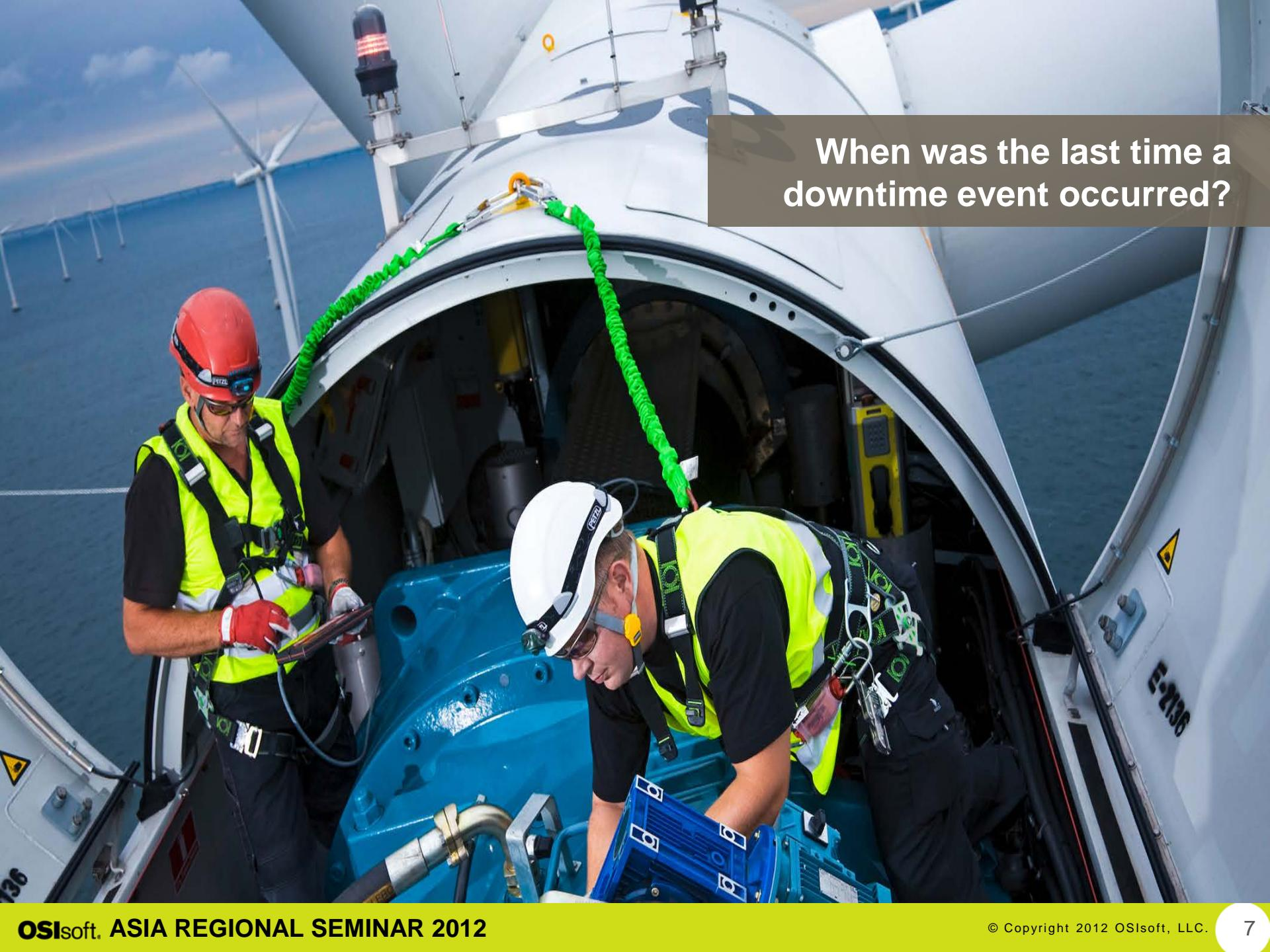
A photograph showing two workers in safety gear (hard hats, high-visibility vests, and harnesses) performing maintenance on the interior of a wind turbine nacelle. One worker is standing and holding a tool, while the other is crouching down. The nacelle is white, and the interior is blue. A green safety lanyard hangs from the ceiling. In the background, several other wind turbines are visible against a cloudy sky.
