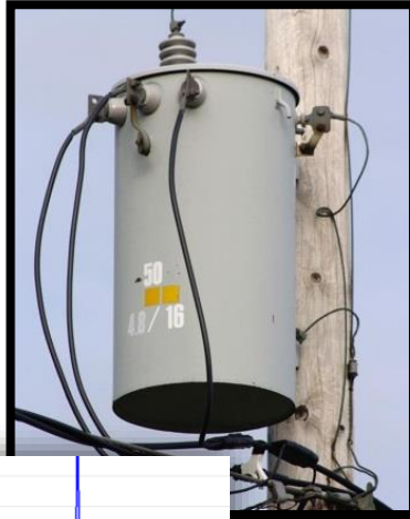
Failing Pole Top Transformer
