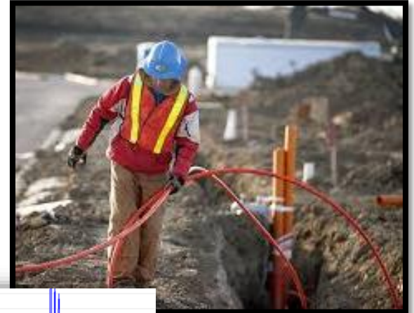
Failing Underground Cable
