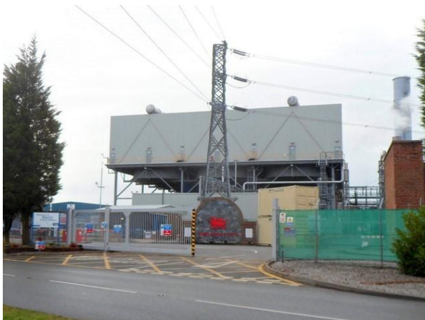
Barry Power Station
