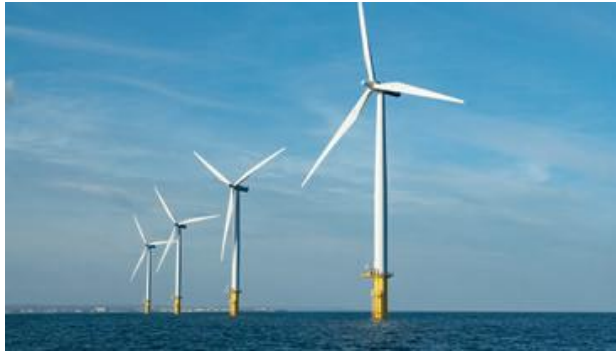
Wind Turbine onshore & offshore
