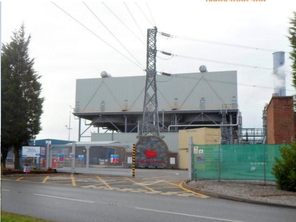
Barrs Power Station
