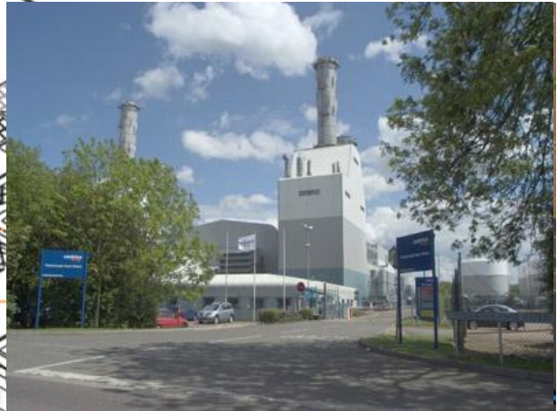
Petton Gas Reception Station
