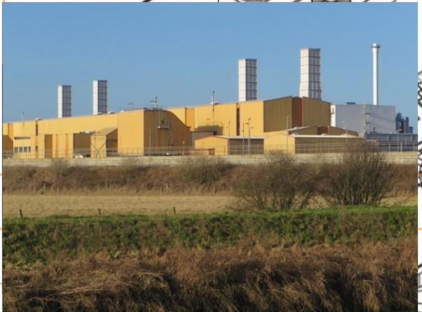
Roby Power Station
