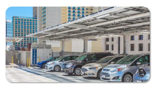
120kW / 615kWh battery 50kW solar PV EV charging 3<sup>rd</sup> floor microgrid
