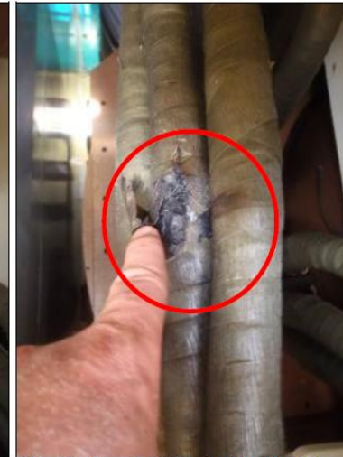
Photo 8 – Burned and Carbonized Lead Insulation
