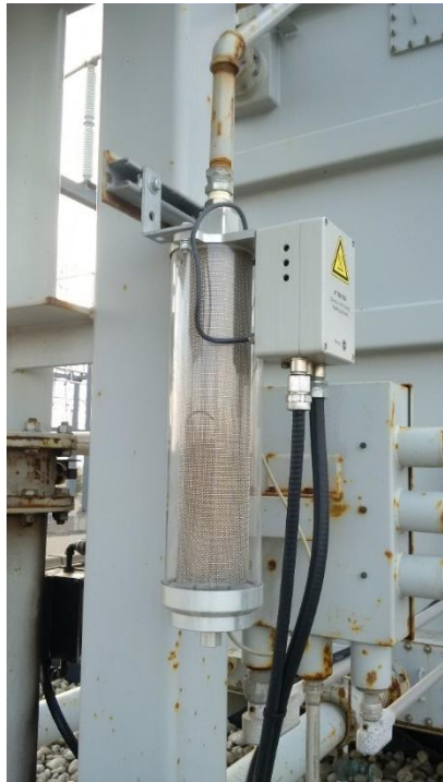
Transformer Self Drying Breather
