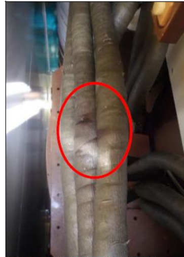
Photo 7 – Discolored Lead Paper Insulation
