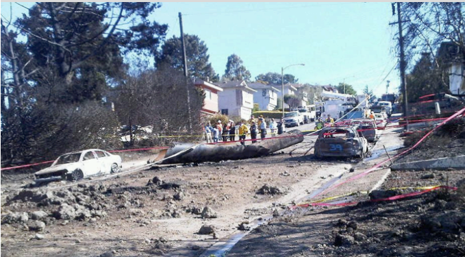
By Bryan - cropped from Close Up Pictures of Gas Line Explosion Damage, CC BY 2.0, https://commons.wikimedia.org/w/index.php?curid=11465628
