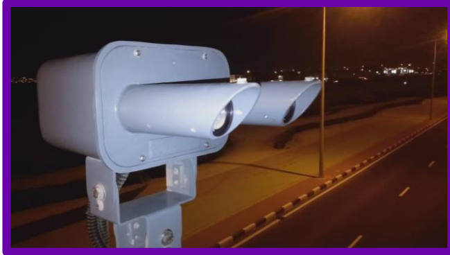
8+ Over Height Detection System (OVDS)
