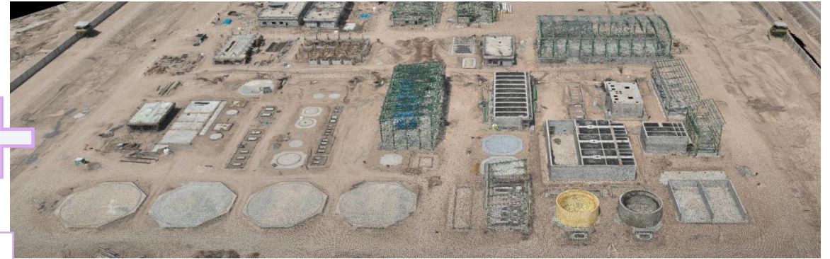
Actual Site Survey By Drone
