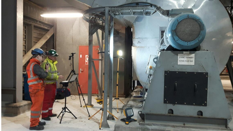
Typical Induced Draft Air Fan
