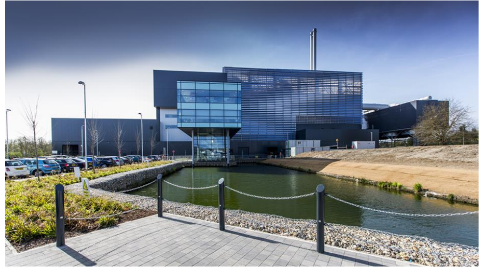
Suffolk Energy from Waste Plant
